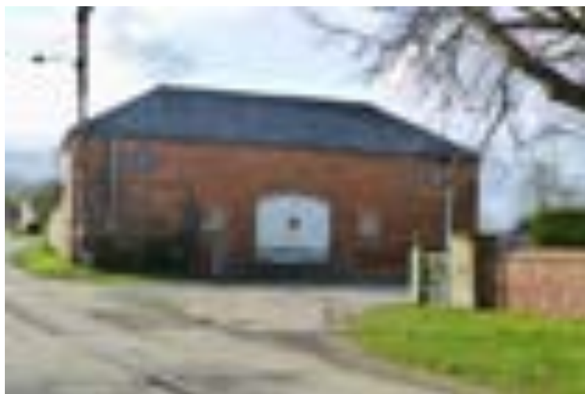
19 th century brick barn (view from Smooting Lane corner)
