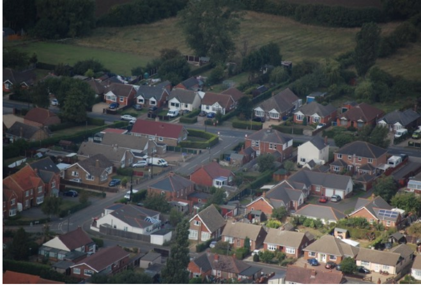
Aerial view of Hawthorn Avenue with the Reepham bungalows along the top of the photograph
