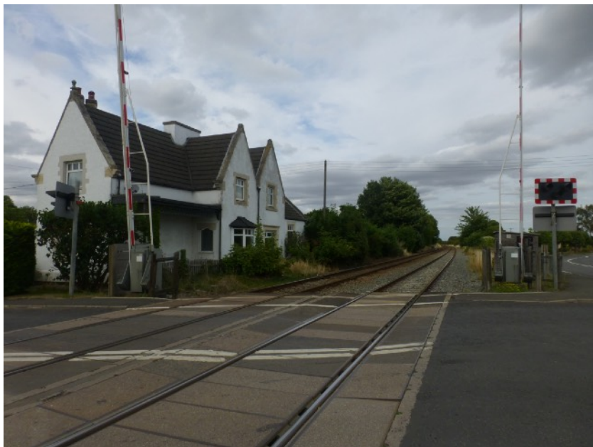
The railway line with Station House on the left - Fiskerton Road begins to the right.
